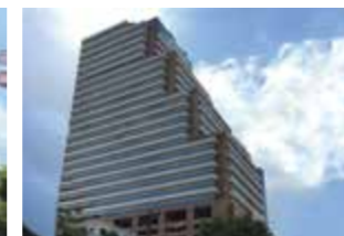
Fujitsu General (Thailand) Co.,Ltd. Bangkok Office (Thailand)
